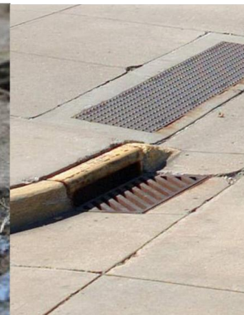
Drains and Catch Basin
